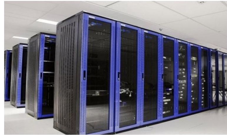
Main Control Room
